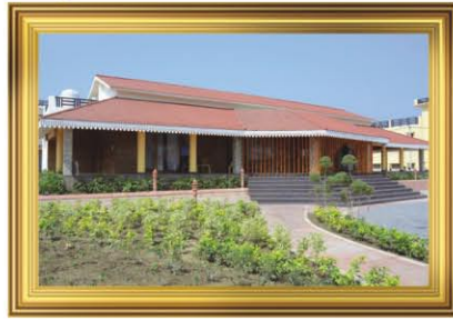
Inspection House, Irrigation Dept., Bazpur
